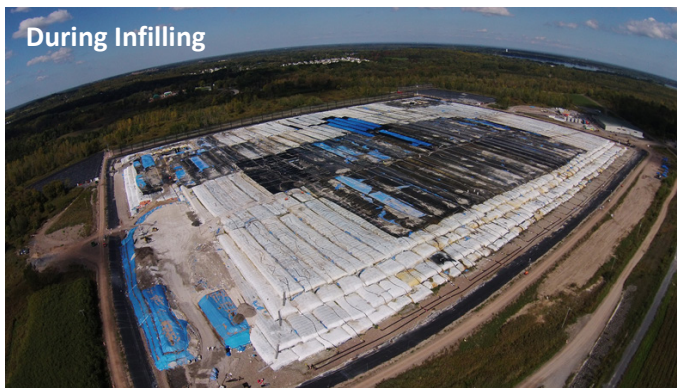
Figure 3: Dredged Material Management Using Geotubes in Upland SCA
