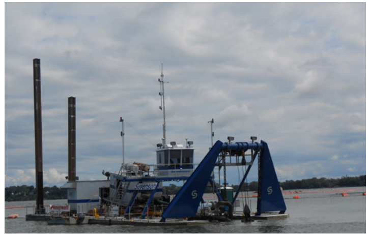
Figure 2: Hydraulic Dredging in Progress
