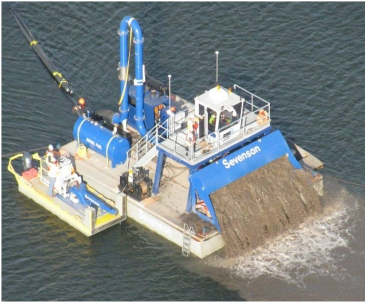
Figure 6: Hydraulic Capping Spreader Barge
